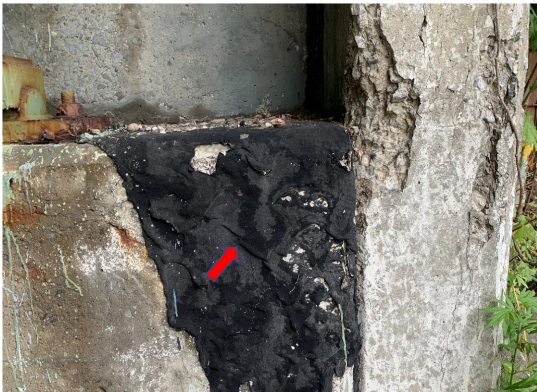
Photograph 6 – View of non-ACM black tar sealant on bridge abutment underside lower half (ACM-11 & ACM-12)
