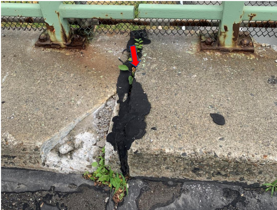
Photograph 3 – View of non-ACM grey foam with black tar sealer on bridge deck (ACM-5 & ACM-6)
