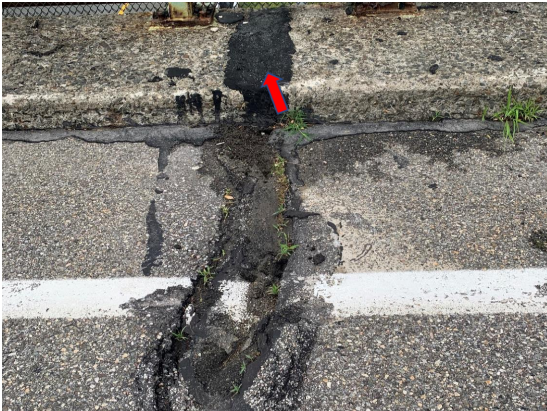
Photograph 1 – View of non-ACM black tar sealant on bridge deck curb (ACM-1 & ACM-2)
