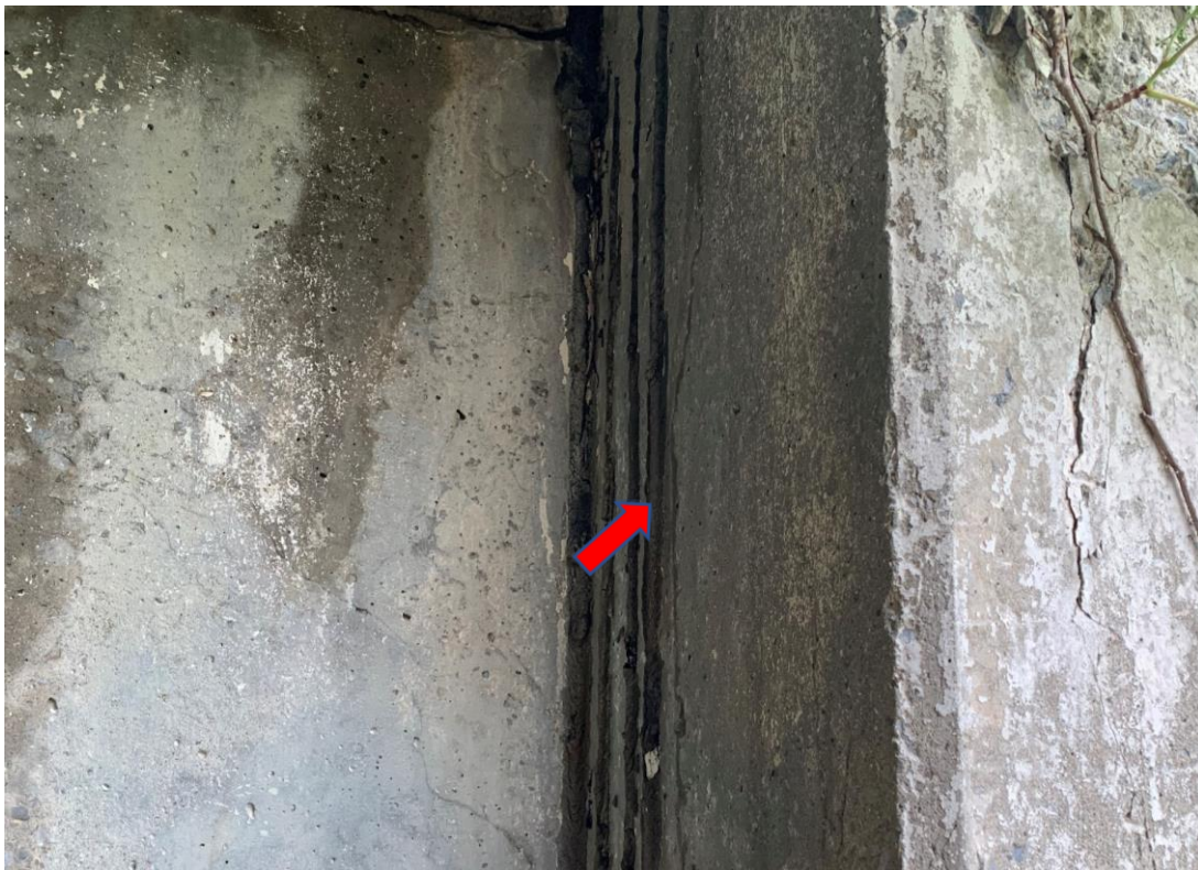
Photograph 5 – View of non-ACM black tar sealant on bridge abutment underside top part (ACM-9 & ACM-10)
