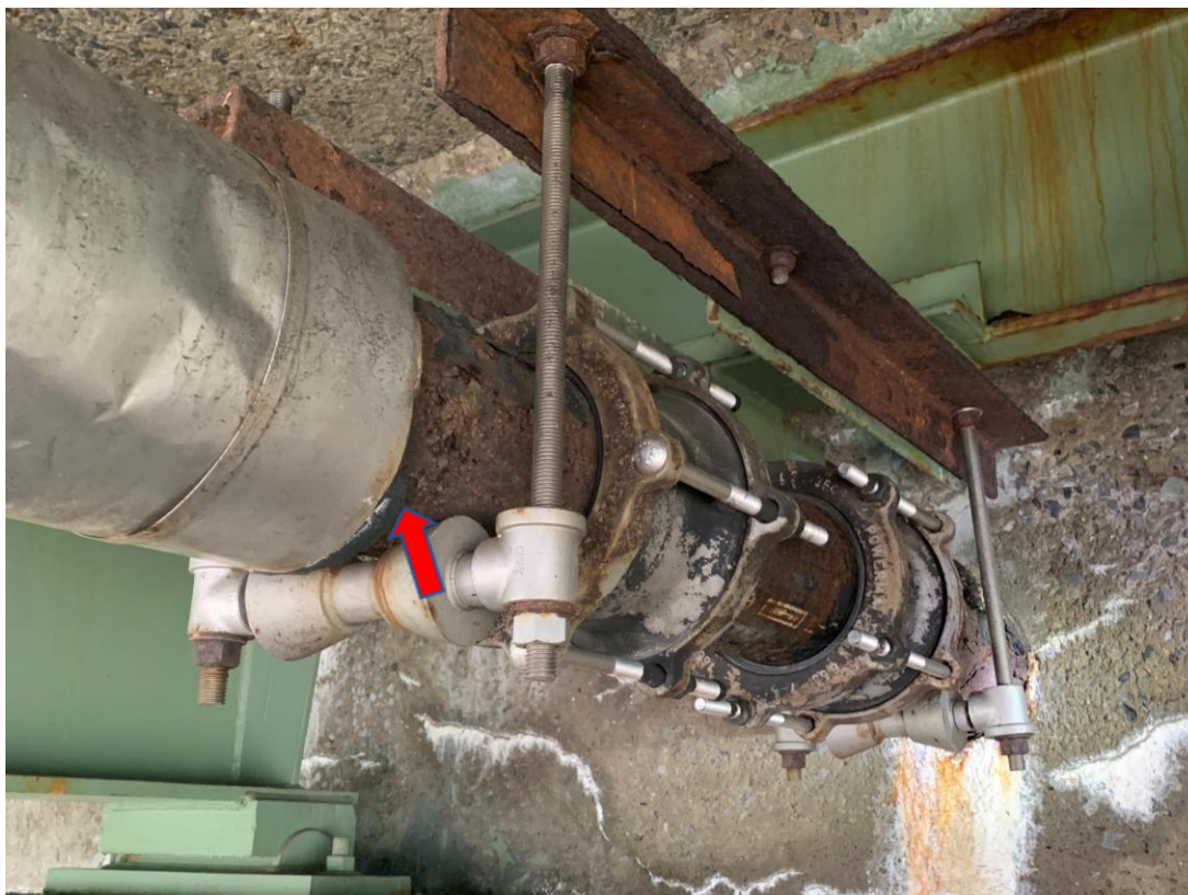
Photograph 4 – View of non-ACM black pipe insulation material from utility pipe under bridge (ACM-7 & ACM-8)
